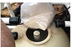
It is recommended that the sand be changed every 5 years to ensure that your pool is maintained in a healthy pristine *condition.* When filter efficiency is allowed to diminish the pool becomes harder to look after and more expensive to run. Water quality becomes a problem due to the inadequate filtration causing chemical usage to escalate.
